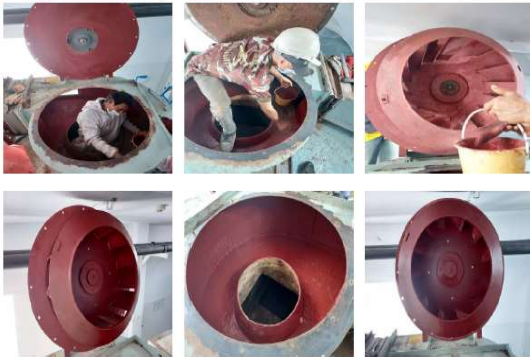
Painting Line2Booth1 (After)
