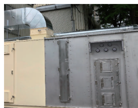
VOC gas activated carbon adsorption system VOCガス活性炭吸着方式
