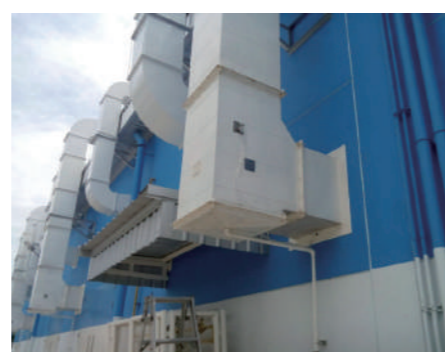
VOC gas Ozone deodorization system VOC gas deodorization method VOCガスオゾン脱臭方式/VOCガス減臭方式
